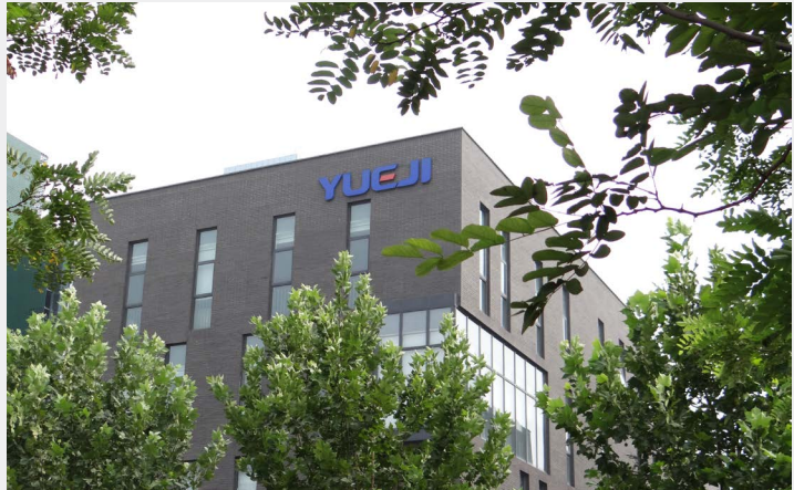
约基总部大楼 The headquarters of YUEJI
